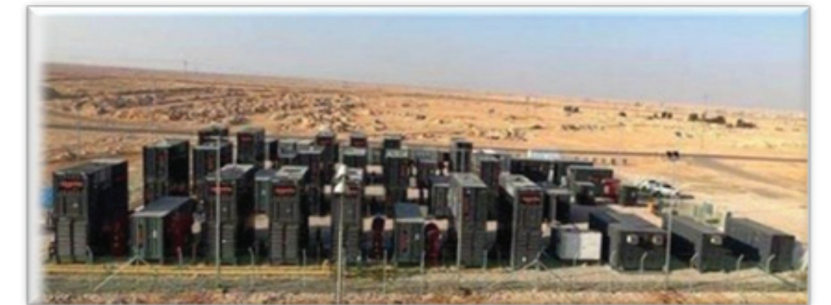
Installation of hybrid power systems to drive a Sucker Rod Pump.
