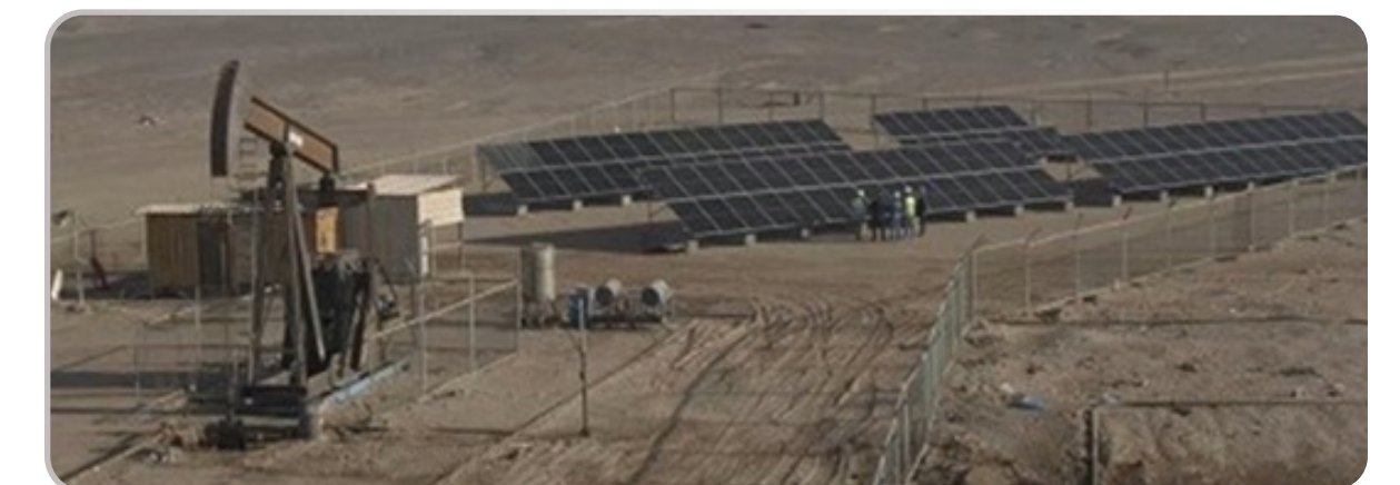
Installation of hybrid power systems to drive a Sucker Rod Pump.
